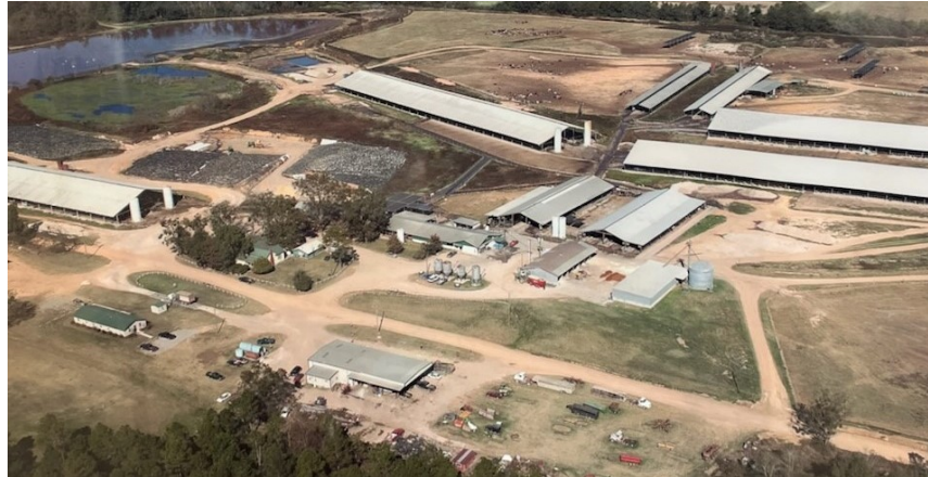
Aerial view of one location showing milking parlor (center), free stall and feed barns (perimeter), silage mounds (left), and outbuildings.
